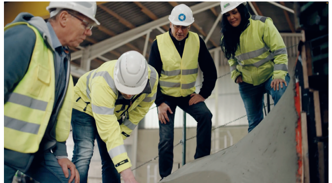
Production of a CO 2 -reduced staircase using a combination reinforcement with the Stabils steel fibre. The fresh concrete with a steel fibre content of 30 kg/m 3 can be easily installed in the formwork.
