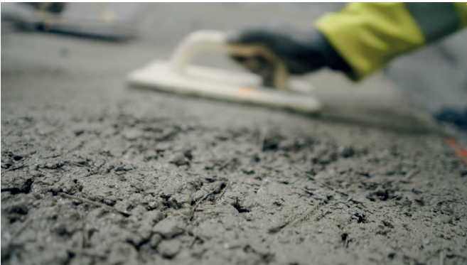
Production of a CO 2 -reduced staircase using a combination reinforcement with the Stabils steel fibre. The fresh concrete with a steel fibre content of 30 kg/m 3 can be easily installed in the formwork.
