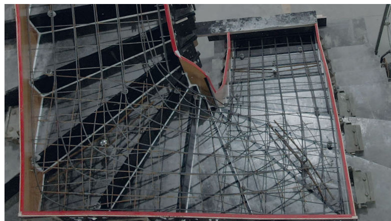
The use of steel fibres supports resource-efficient construction methods. On the left a staircase with conventional reinforcement, on the right a staircase with a combination reinforcement with the same performance characteristics.
